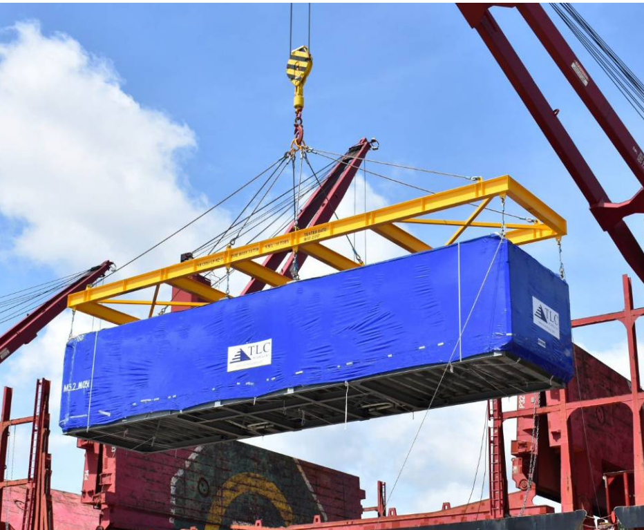
↑ Volumetric construction being delivered to site
